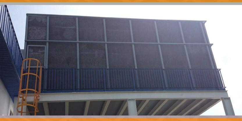
FORTESHIELD aluminium foam panel is a newly-conceptualised metallic material foamed through the melting of aluminium ingot with various chemical components. The texture of the aluminium foam resembles that of a sponge, made up of multi-cell like structure.
